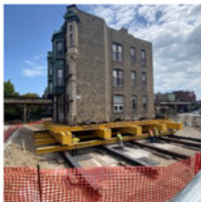
CTA Red-Purple Line Modernization
