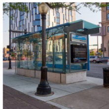
CTA Grand, Chicago, and Division Blue Line Stations Renovation
