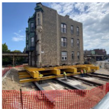
CTA Red-Purple Line Modernization
