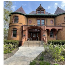
Evanston History Center Restoration
